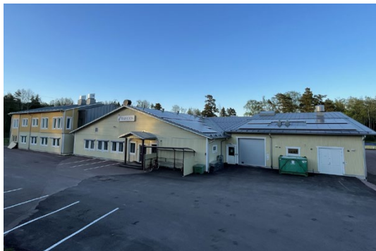
Main building for production & offices with the new solar panels on the roof, INFICON Aaland (FI)
