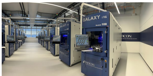
Vacuum gauge calibration systems, Balzers (LI)
